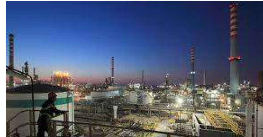
Eni S.p.A., Gela Oil refinery
