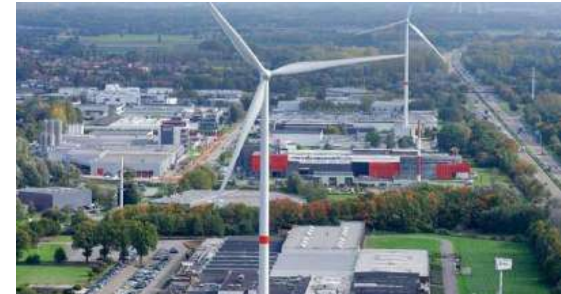
Azteq/Avery Dennison, Turnhout Adhesive manufacturing plant 1
